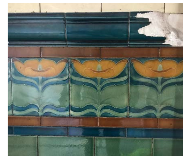
Close up of the Pilkington tiles in the Cocoa Rooms, 2018 © Julian Harrap Architects LLP
